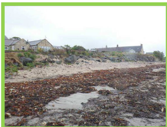
New rock revetment toe now well vegetated (/2601C03) – constructed May 2016
