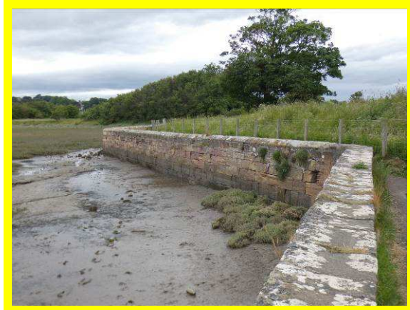
Masonry wall fronted by salt marsh (/2801C06)
