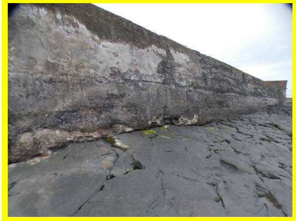
Front face of Pier (/2201C11)
