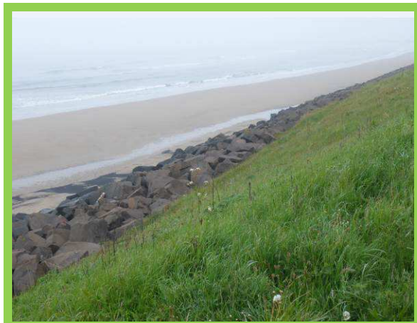
Rock revetment protecting former foundry site (/3901C05)
