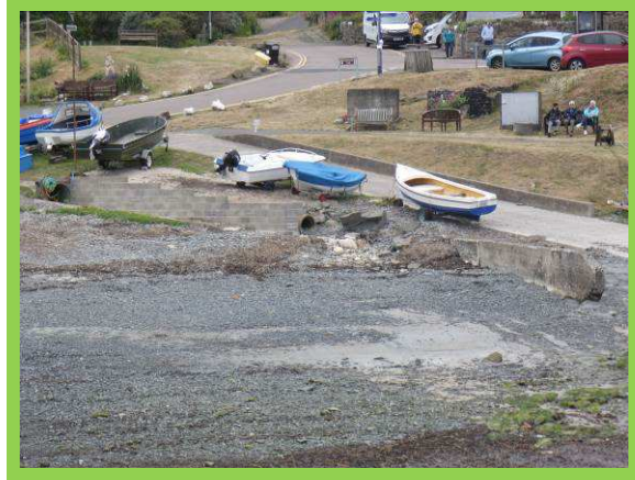
New blockwork wall (/2201C06)
