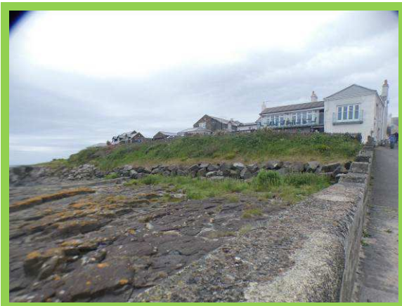
Inactive slopes with rock revetment at toe (/2201C13)
