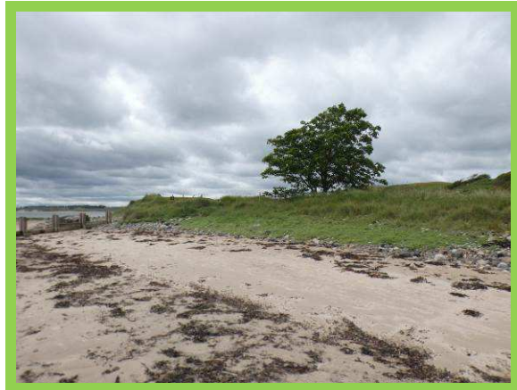
Isolated timber groyne (/2701C04)
