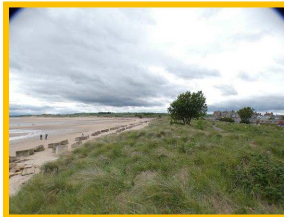
Severe erosion extending beyond two rows of tank blocks (/2701C08)
