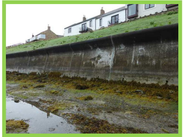
1701/C18 Wall and slope in good condition
