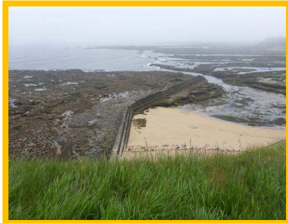
Green's Haven Breakwater remains in poor condition but still retains beach sand (/0701C04)
