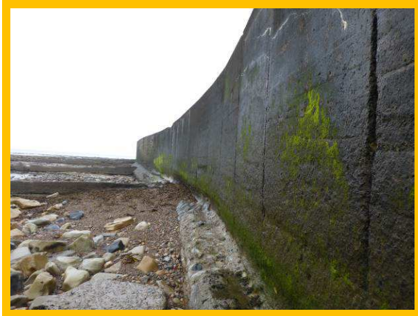
Landward section of Blyth East Pier (4001C04)
