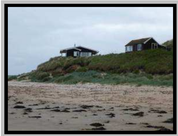
Previous dune damage followed by recovery at Newton Haven (/2001C03) 2016
