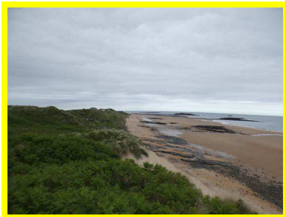
General erosion of dunes (/2001C03) 2018
