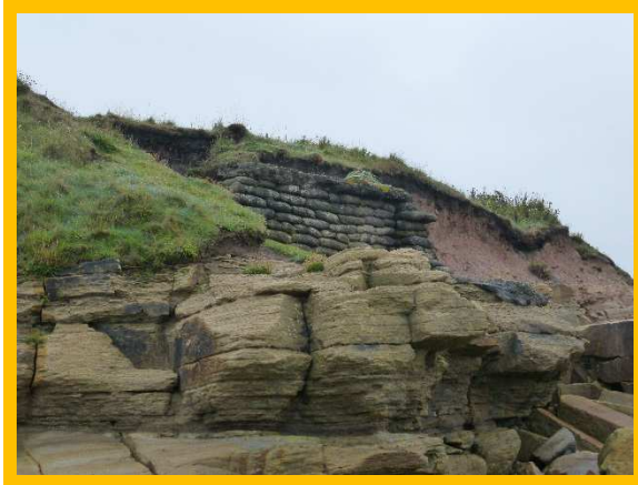
Ongoing erosion of cliffs around Dell Point (/1701C28)
