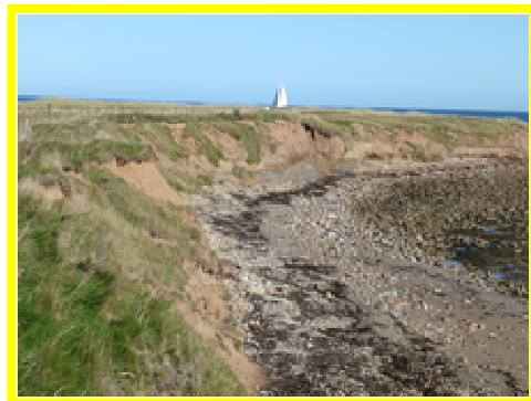
Erosion of soft cliffs remains an ongoing process (/5001c04).
