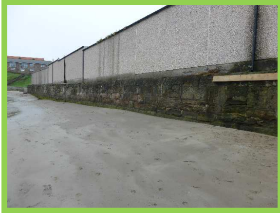
1701/C15 Good condition
