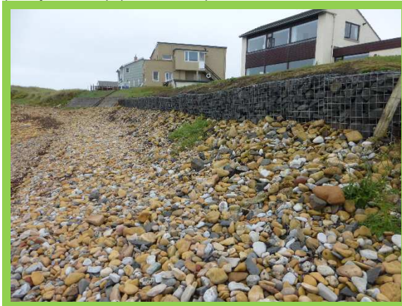
New gabion basket wall in good condition. (/1701C41)
