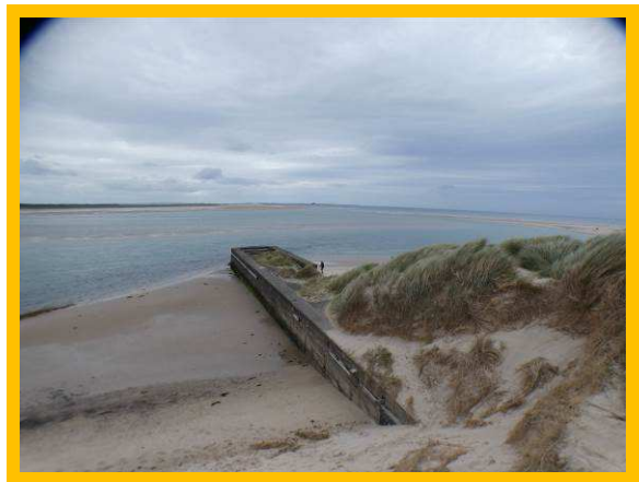
1501/C06 – south face and core of jetty
