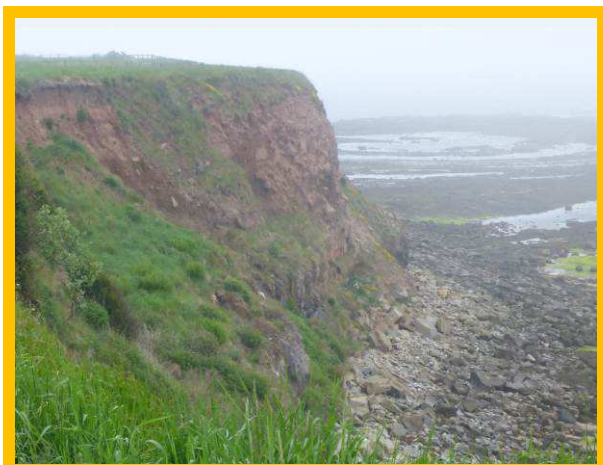
Slumping cliffs along Magdalene Fields Golf Course (/0701C12)
