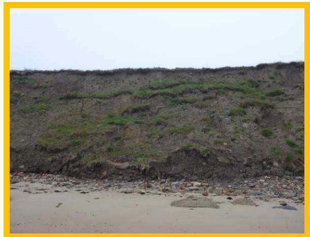
Eroding cliffs south of Cambois House (/3901C01)
