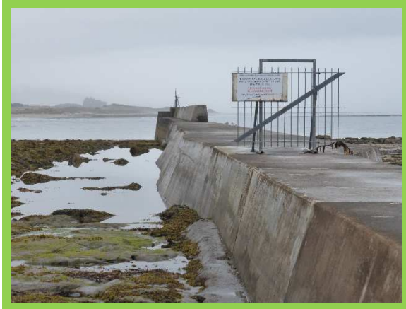
1701/C20 No signs of damage
