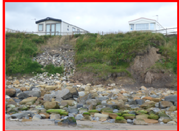
Erosion recommences to immediate south of rock berms (/3701C03)
