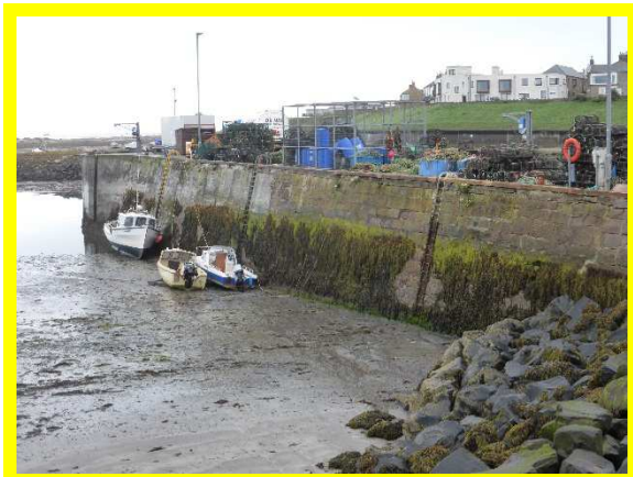
Inner face of the Inner Pier 1701/C10
