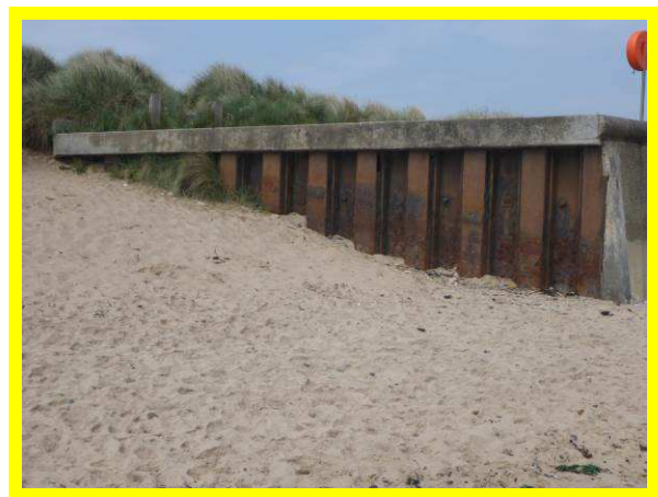
Steel sheet pile end to promenade (4201C08)
