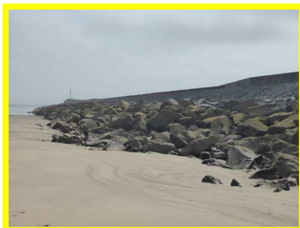
Rock armourstones on north face of North Pier (/3001C01)
