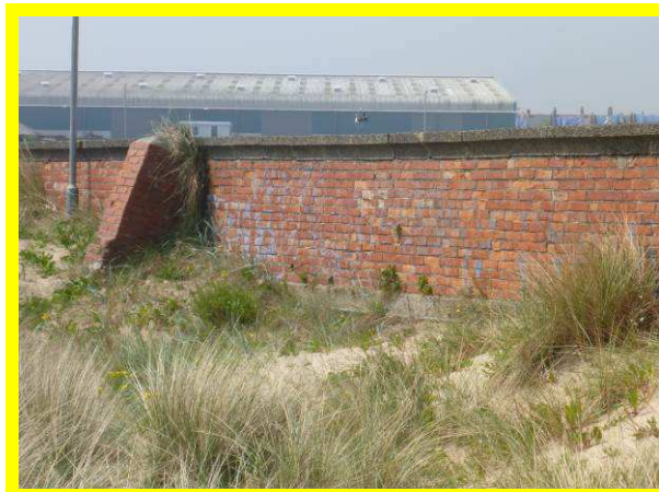
Masonry wall to rear of dunes (/4201C10)
