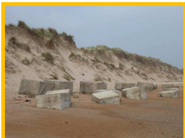
Due erosion in central South Bay (/4301C02)
