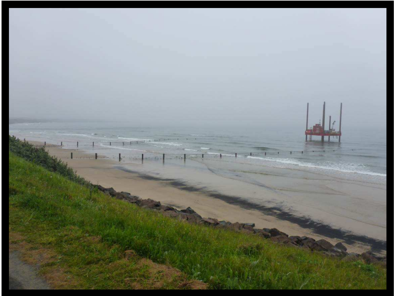
Cable landfall works for North Sea Interconnection (/3901C05)
