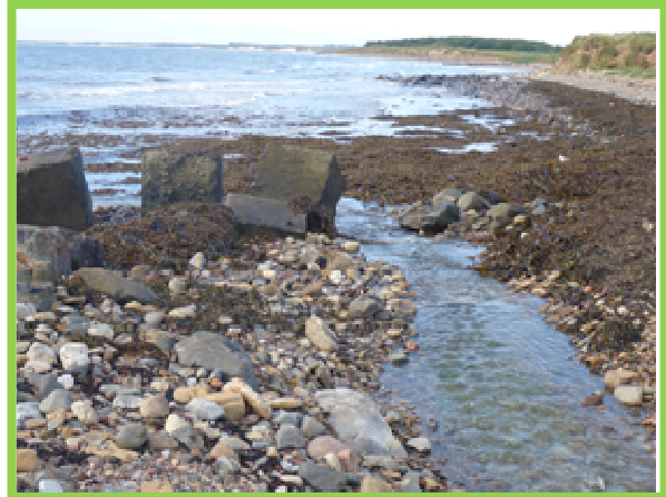
Drainage occurring alongside of remnant outfall structure through gravel, cobbles and boulders (/3201C09)
