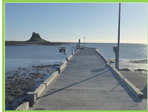
Improvement works to harbour pier (/4901c09)
