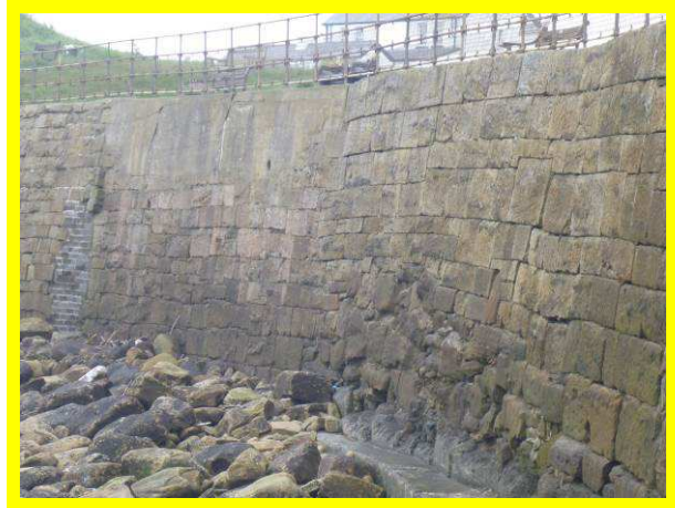
High masonry wall (/4401C11)
