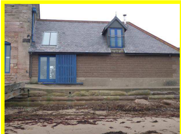
Wall in fair overall condition (/0801C05)
