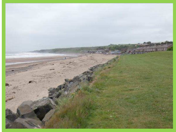
1001 c01 – 2018 showing increased beach width with groynes buried.
