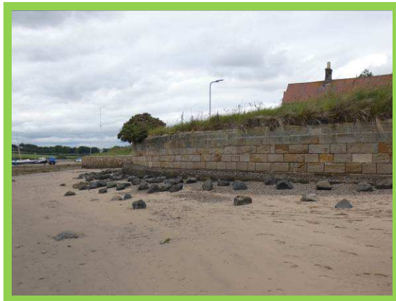
Masonry wall with concrete and cobble toe apron (/2801C02)
