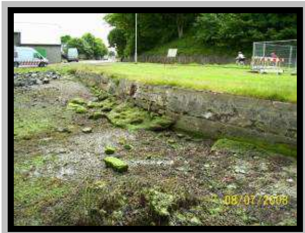
901c05/06 in 2008 showing toe level and condition of masonry.
