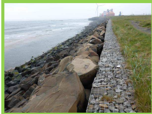
Rock revetment and gabion baskets (/4001C01)
