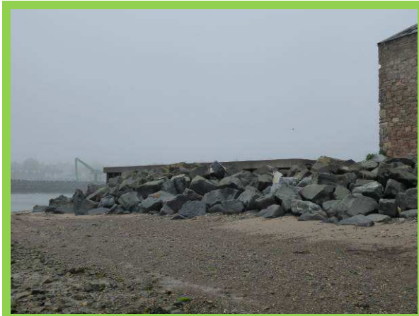
Rock revetment in good overall condition (/0801C04)
