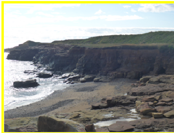
Currently relatively stable cliffs around Beacon Point (/3501C03)
