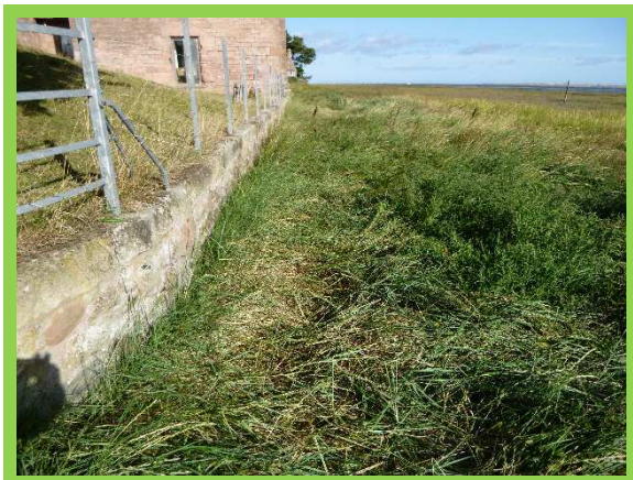
1401/C23 – local defence north of slipway.
