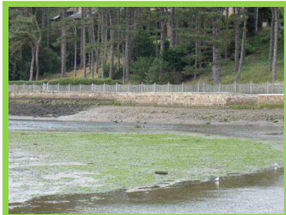
Footpath repaired wall (/2801C10)
