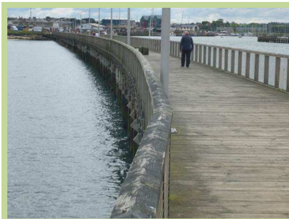
South Jetty in good overall condition (/3001C11)
