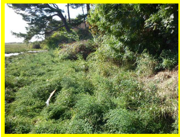
1401/C23 – dense vegetation covering the local timber defence.
