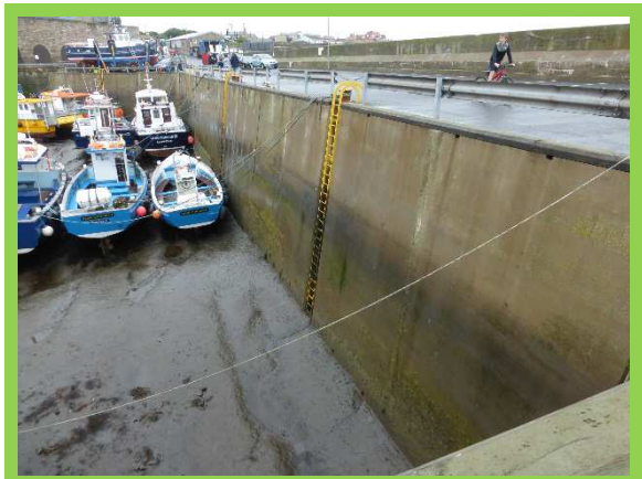
Inner face to North Pier 1701/C11
