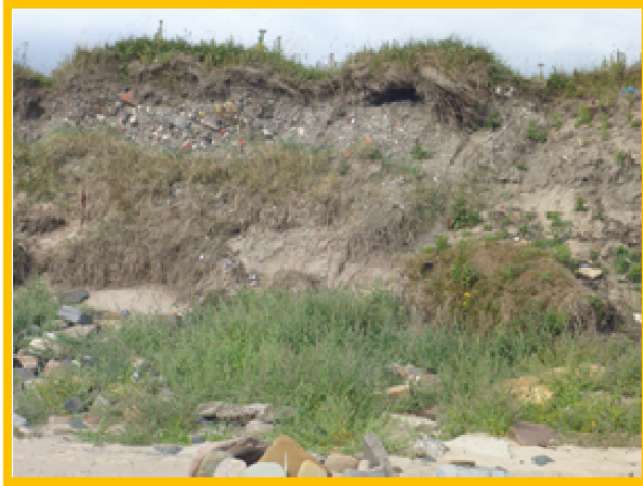
Active slumping at northern section fronting caravan park (/3501C05)
