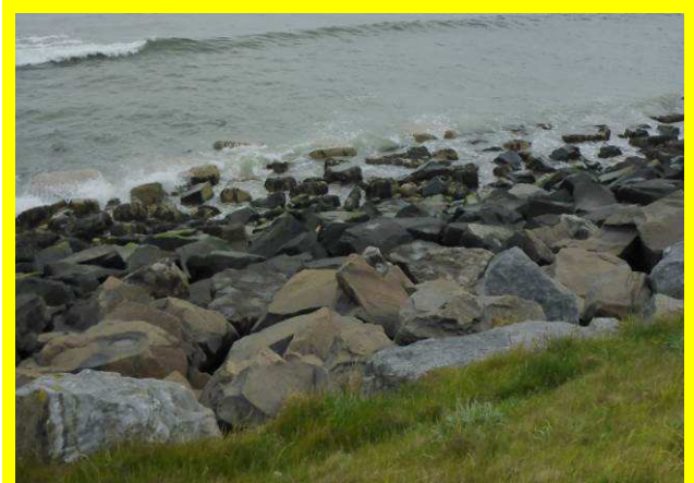
Composite defence with timber breastwork (/4001C02)
