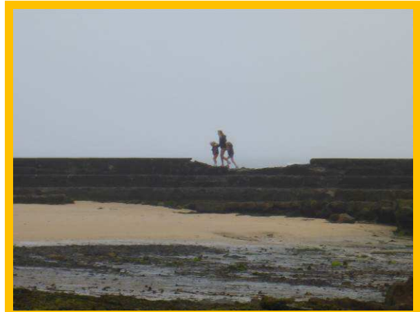
Adult and two children on breakwater crest in damaged section (/0701C04)
