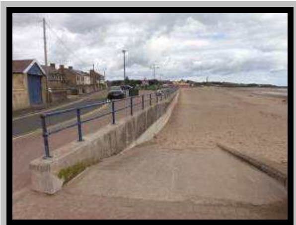
1001 c02 – high beach levels with good crest width 2016.
