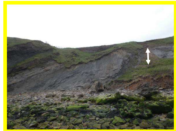
1001 c05 – slight slippage 2018.
