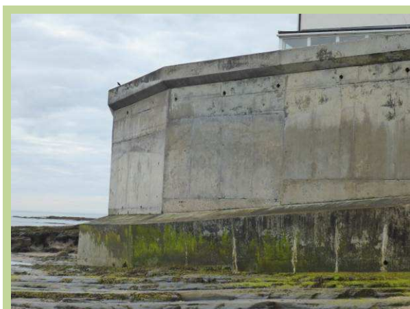
Substantial seawall in overall good condition (/3101C07)
