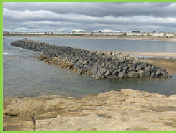
North breakwater in Newbiggin Bay in overall good condition (/3601C13)
