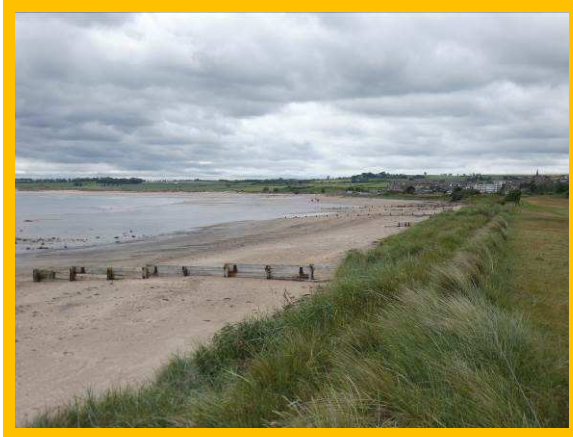
General exposure of timber groynes (/2701C05)
