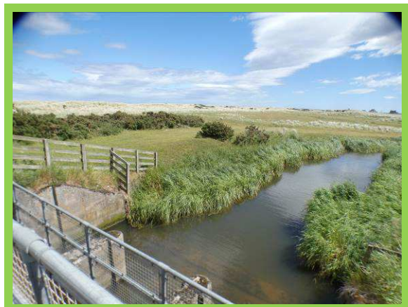
1301/ C01, North Low sluice
