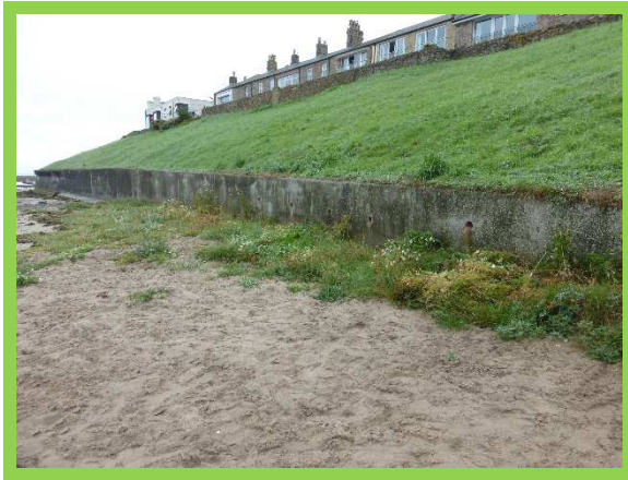
1701/C17 Good condition
