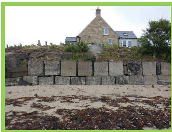
Stacked concrete blocks (original scheme) with rock revetment (2013 (emergency scheme) (/2601C02)
