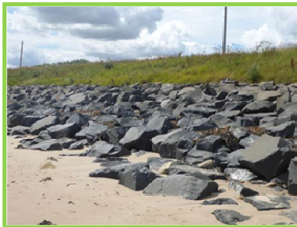
Wide rock revetment in good condition (/3201C03)
