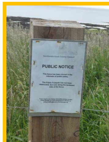
Relocation of fencing and footpath due to slumping cliffs along Magdalene Fields (/0701C12)
