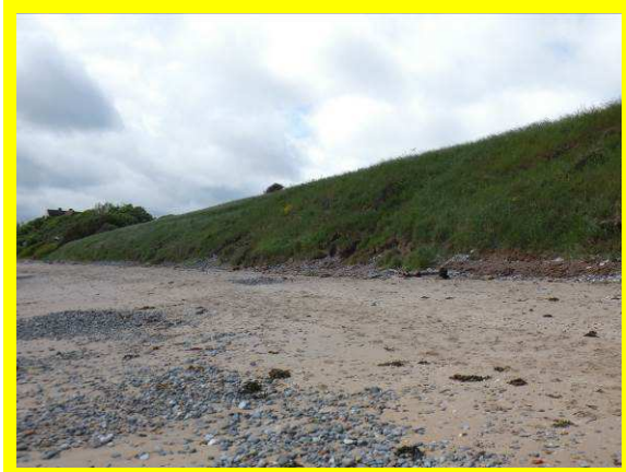
Stable and well vegetated slopes near Foxton Hall (/2701C02)
