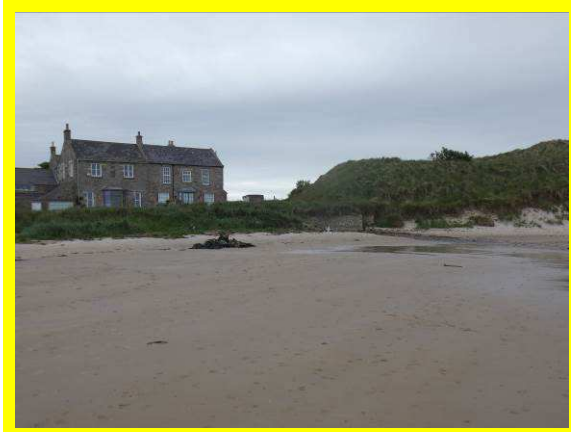
Some minor erosion around Monk's House but not significant risk 1601/C03
