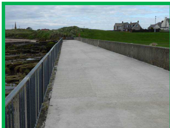
Promenade deck remains in very good condition following previous repairs (/3101C05)
