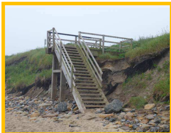
Erosion of cliffs near recently-installed access steps (/3901C03)
