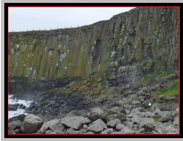
Localised rock fall at Castle Point (/2001C05) 2016
