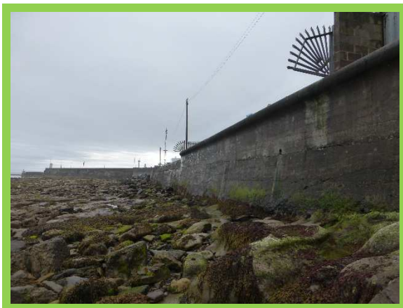
Harbour wall in good condition 1701/C05.
