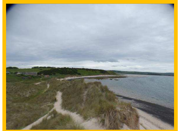
1501/C06 – 2018 major area of erosion to south of jetty
