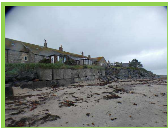
Stacked concrete blocks (original scheme) and rock revetment (emergency scheme) at southern end of Boulmer village (/2601C05)
