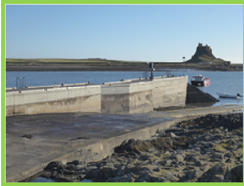
Improvement works to harbour pier (/4901c09)
