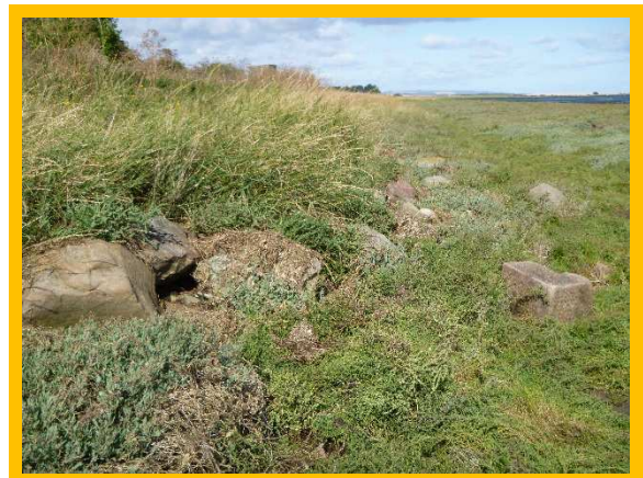
1401/ C23, vegetation covering localised rock defence
