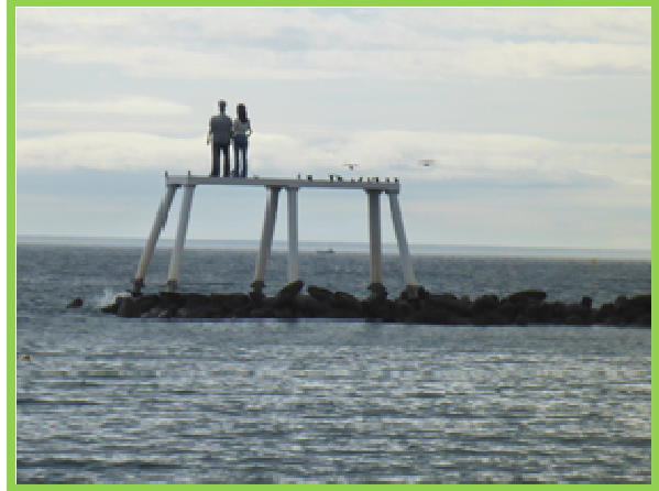
Detached breakwater in central Newbiggin Bay remains in very good condition with salient/tombolo developed in lee (/3601C13)
