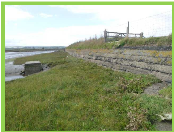
1401C14 – Concrete block revetment and outfall in good condition
