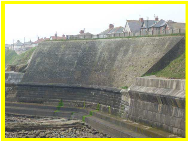
Seawall with upper brickwork retaining wall (/4401C15)
