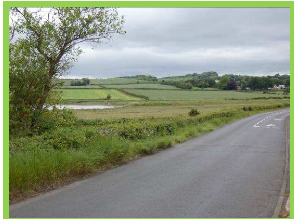
Area of realignment (/2801C11)
