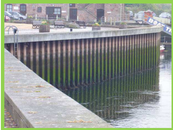
Steel sheet piled quay walls in good overall condition (/0801C03)
