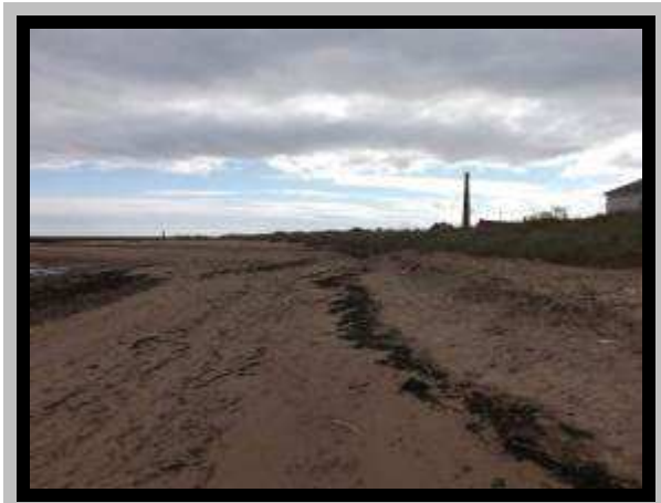
901c08 – cliffing and erosion 2016.
