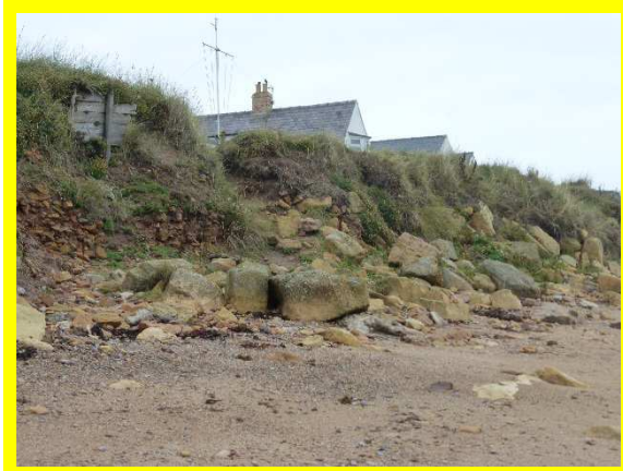
Ongoing erosion to slopes fronting properties (/1701C44)
