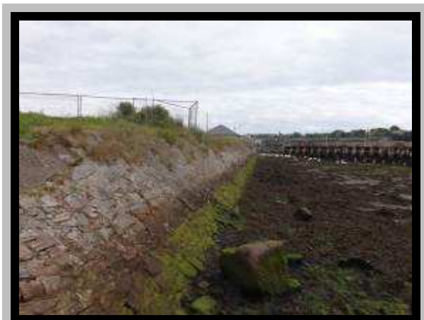
Masonry revetment 901c04 at northern end -2016.
