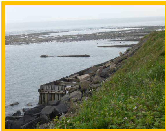
Composite defence with timber breastwork (/4001C03)
