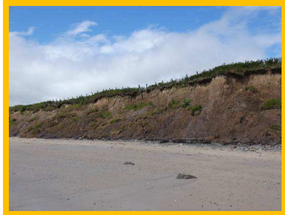
Cliff failure affecting a long section of fencing (/2701C01)
