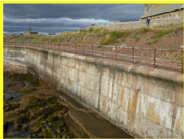
Church Point seawall in fair overall condition (/3601C12)
