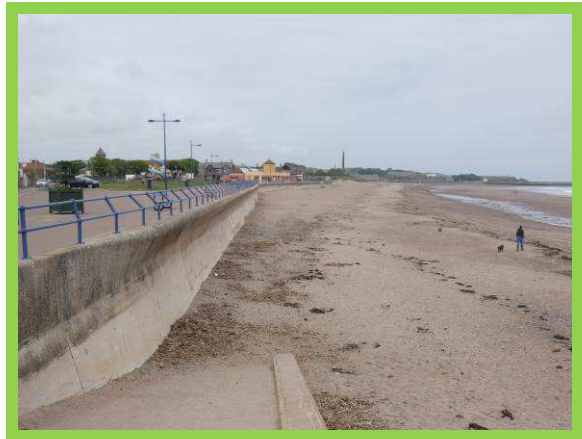
1001 c02 – some reduction in beach levels with realignment of beach shape 2018.
