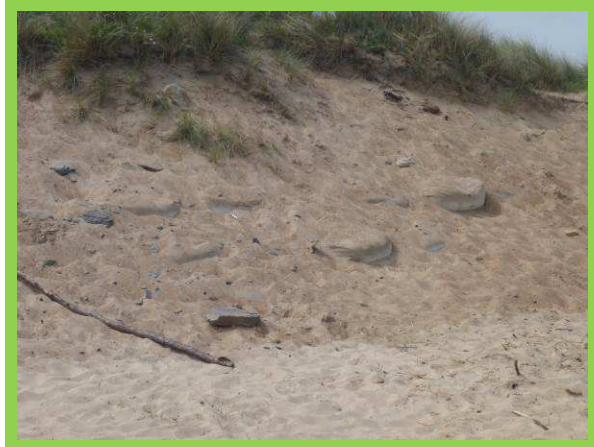
Exposure of sand bags on dunes near Meggie's Burn (/4301C01)
