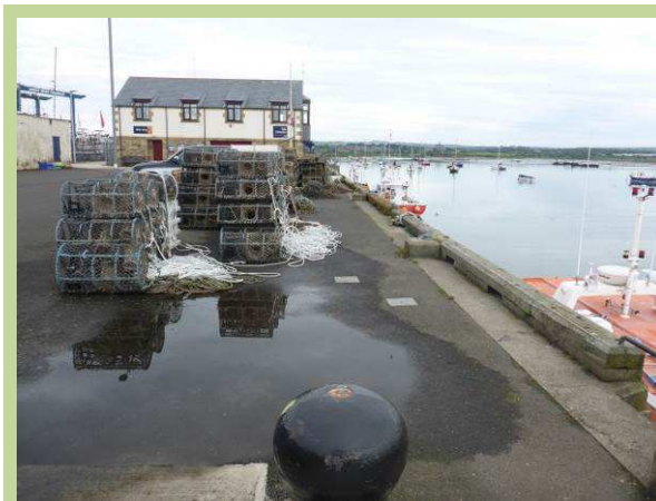
Quay wall in good overall condition (/3001C05)
