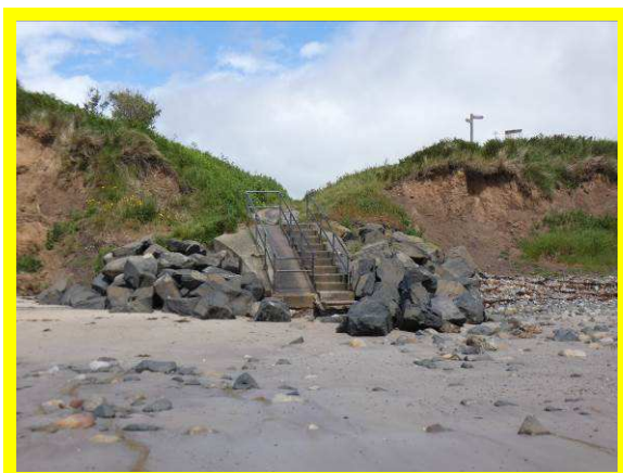
Rock armour around access steps in north of Foxtan Bay (/2601C09)
