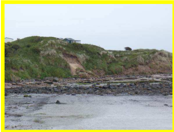
Front face dune failure (/2601C07)
