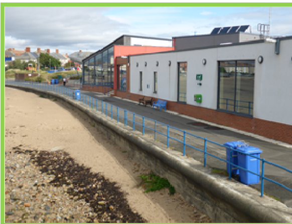
High beach levels and wind-blown sand to rear of promenade in northern sections of Newbiggin Bay (/3601C15)
