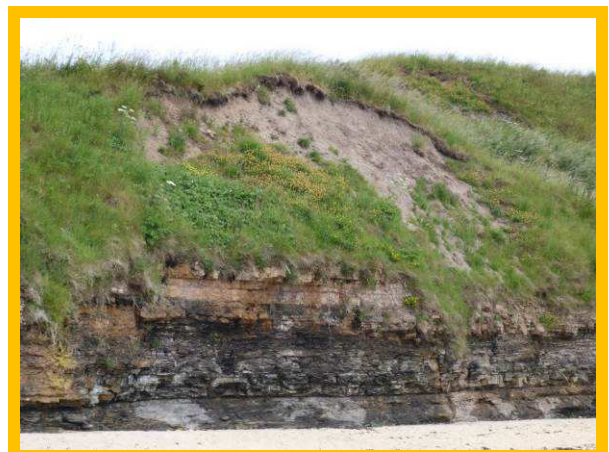
Slumping in cliffs at Greens' Haven (/0701C08)
