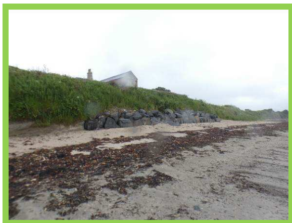
Rock revetment toe to locally protect isolated property (/2601C01) – constructed May 2016, now vegetated above.
