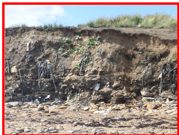
Actively eroding spoil cliff (/3401C05)
