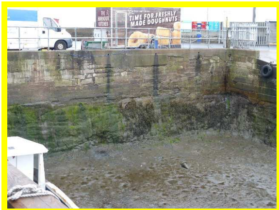
No signs of deterioration 1701/C12
