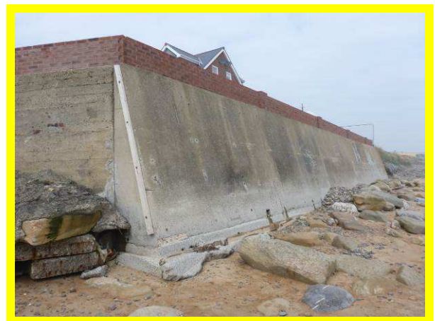
Existing sea wall protecting new properties (/4201C04)
