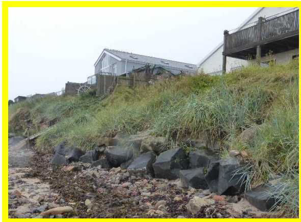
Recently placed rock armour fronting properties at Beadnell Haven. (/1701C24)
