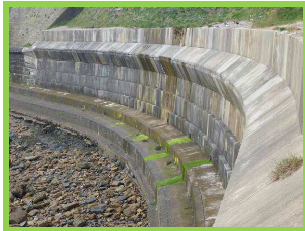
Near-vertical seawall (/4401C14)
