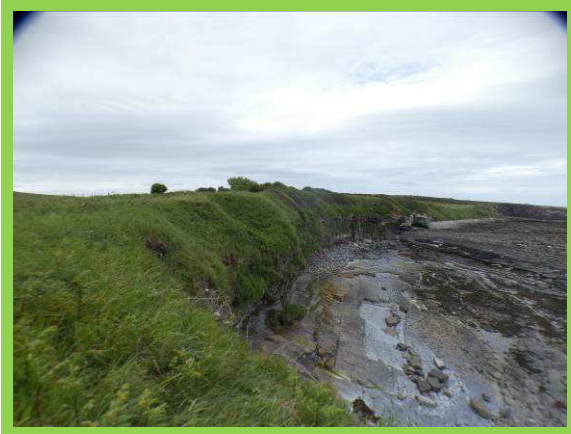
Slow undercutting (/2401C01)
