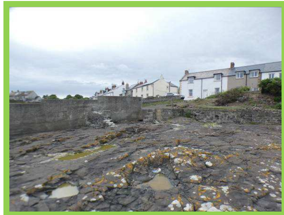
Wall and start of Pier (/2201C02 / C03)
