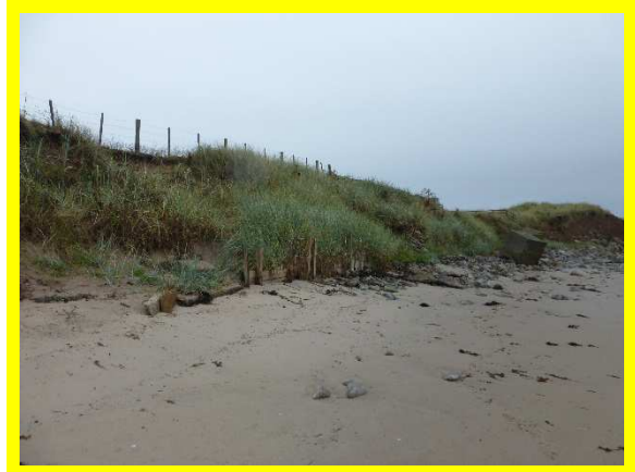
1701/C23 limited erosion to golf course
