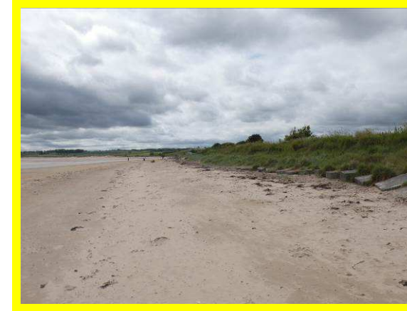
Slight recovery over the southern end of (/2701C06)
