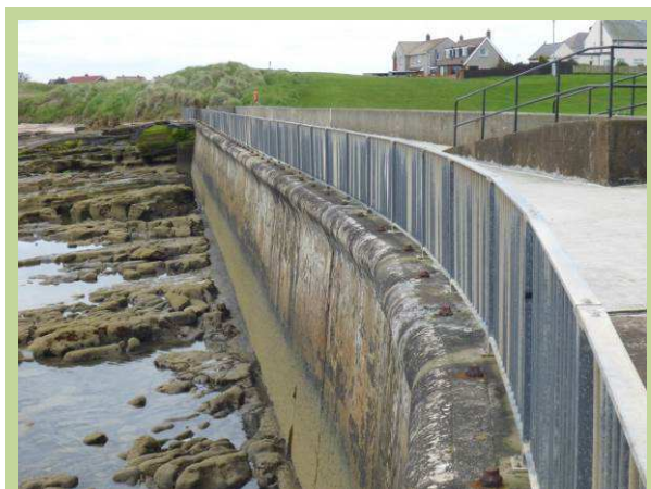
Seawall in good condition despite rust-staining (/3101C05)
