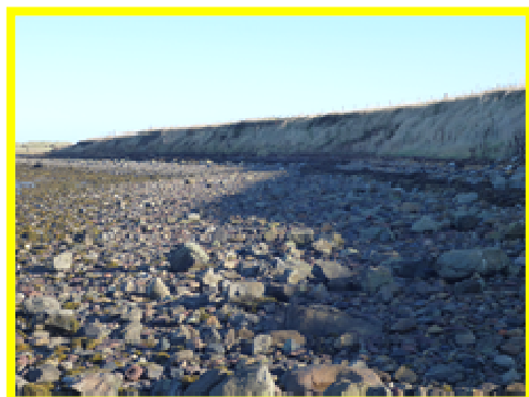
Eroding section of higher cliff (/4901c03).
